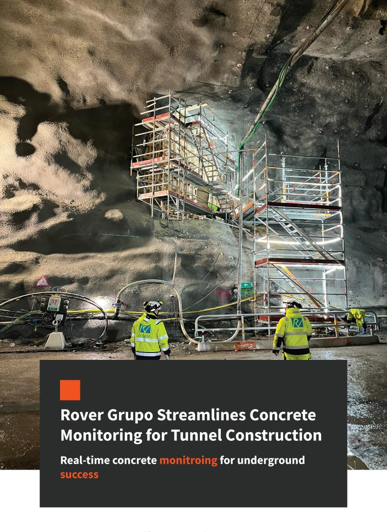
At Rover Grupo Sweden, the decision to implement a sensor-based solution for concrete monitoring has enabled significant improvements in their tunnel construction projects. By choosing an automated system like Maturix over traditional data loggers, Rover has been able to streamline documentation processes and gain better control over the concrete curing phases.
