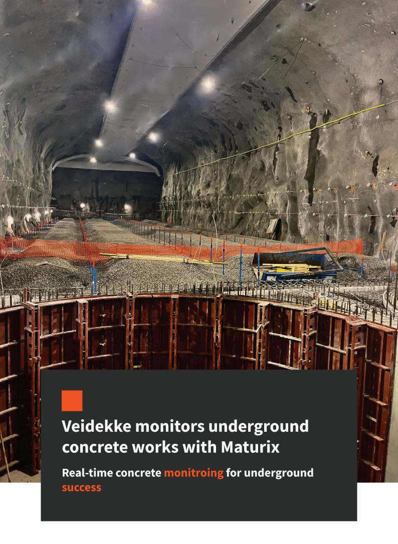
As part of Stockholm's future wastewater treatment system, Veidekke is building new underground structures in rock beneath Hammarbybacken. The work includes extensive concrete elements such as thick roof slabs, where precise timing and clear documentation are essential — particularly when it comes to formwork removal and safety planning.
